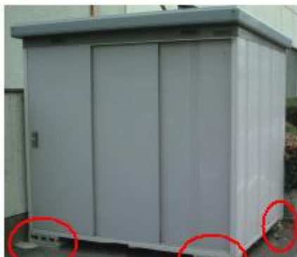
A shed simply put on concrete blocks directly on the ground
